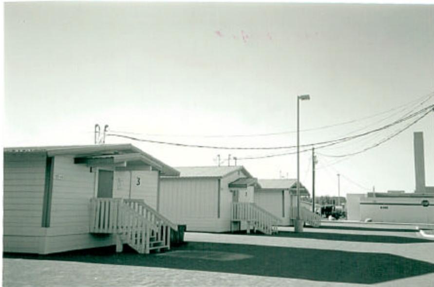
Portable classrooms at Wendler Middle School without ADA access
